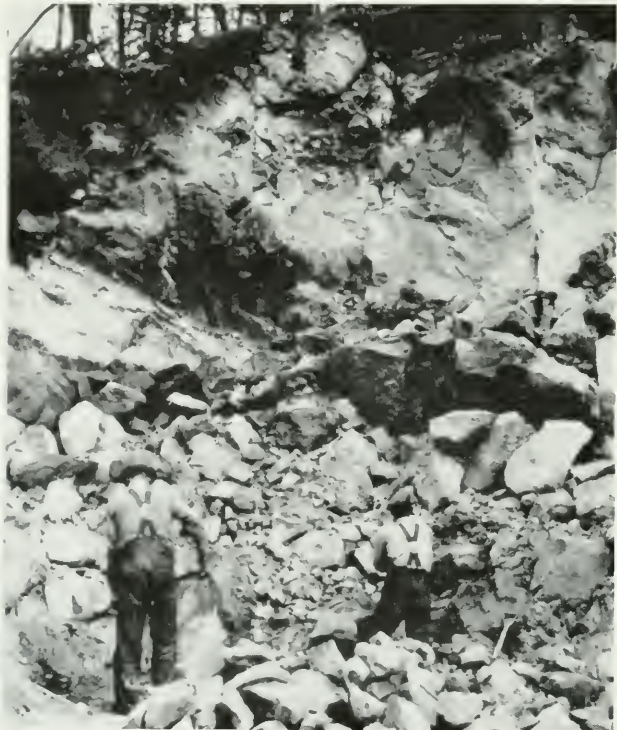
FIGURE B.—Screening out fines in olivine quarry after blast.
